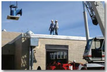
Huntsville Utilities Water Department performs many tasks in-house to keep customer rates down. Pictured above and at right, staff install a high service pump at one of the treatment plants. A crane lowers a part thru a skylight as staff wait to complete the installation.
